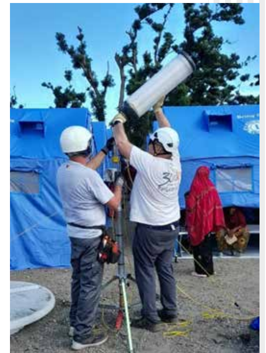
Installation of solar streetlights in emergency shelters in Mayotte
